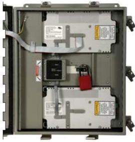
Next-generation SPDs come with safety barriers and lockout/tagout provisions that protect technicians from injury during maintenance procedures.
